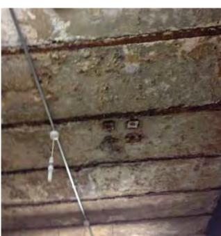
Figure 4.2 - Slab soffit showing evidence of dampness
