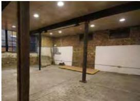
Figure 6.1 – Unusual propping to first floor east wing
